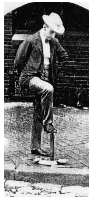
Photo from Sellers' brochure showing what may be the inventor lowering the hitching post into its housing. No warnings were posted regarding children standing over the device and raising it. (Courtesy Kutztown Area Historical Society)
